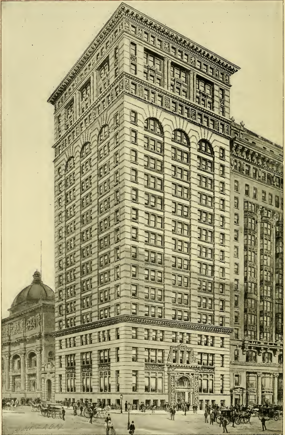
Bank of Commerce Building and New York Clearing House, containing respectively 566 H.P. and 418 H.P. Babcock & Wilcox Boilers.
